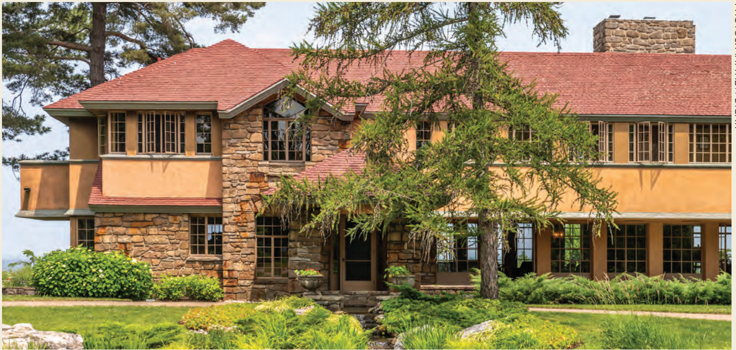
PHOTOS: MATTHEW DIGATI
